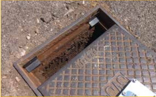
Shims positioning between cover and frame.
