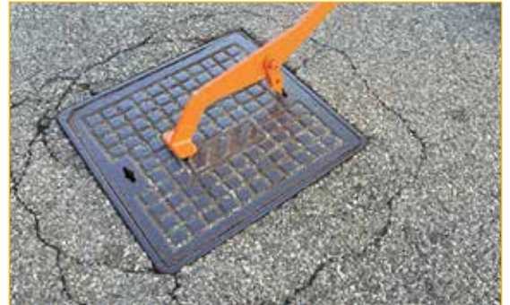
Inserting the hook into the slot and rotate to 90°.
