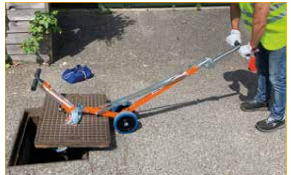
Use 2: opening with wheeled lever APS90 or APS80.
