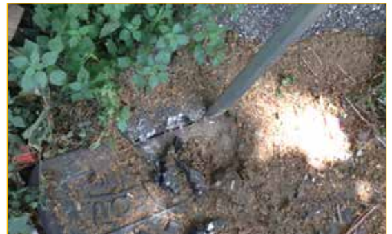
Useful for cutting layers of asphalt and concrete, cleaning and peeling dirt, which often cover the surface and the frame of the lid.
