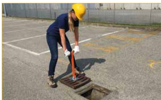
Opening manually light/middle weight lid.
