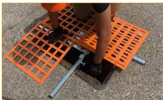
Inspection site opened
